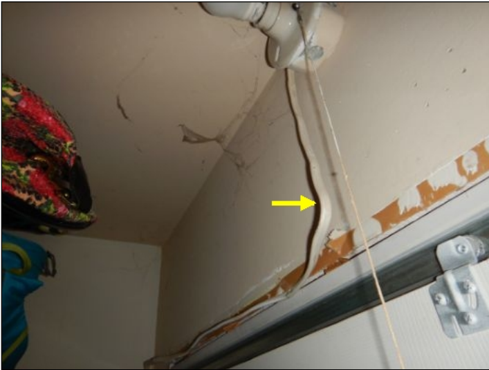
Exposed wire in the Closet of the Master Bedroom below 8 feet and subject to damage [2][4] Unprotected wires were noted within 6 feet of the Attic Access [2][5]
