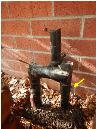
Shut-off Valve for the Main Water Line
