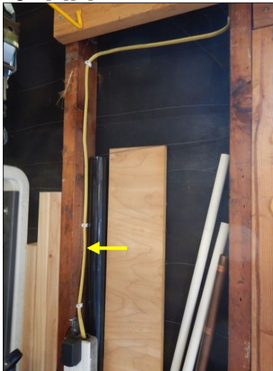
Exposed wires in the Garage were below 8 feet and subject to damage [2][4]
