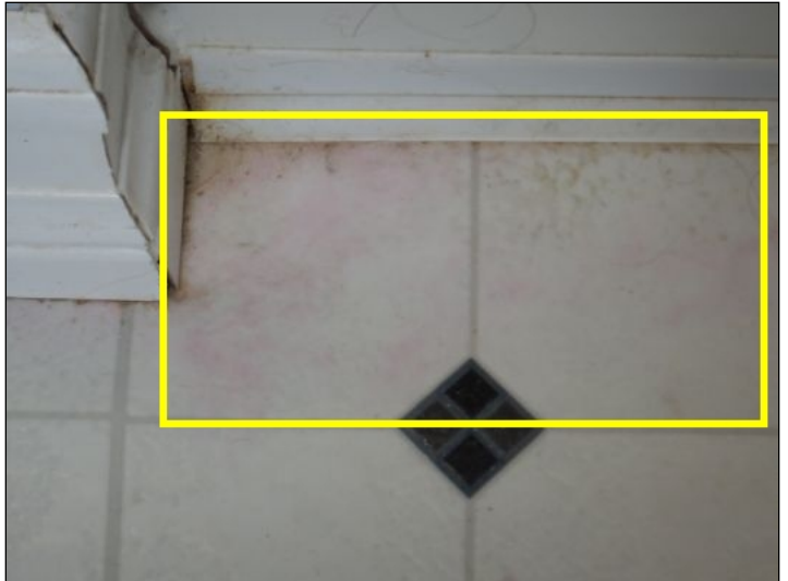
Discoloration of the Vinyl in the Master Bathroom is consistent with moisture being present under the Vinyl [2]
