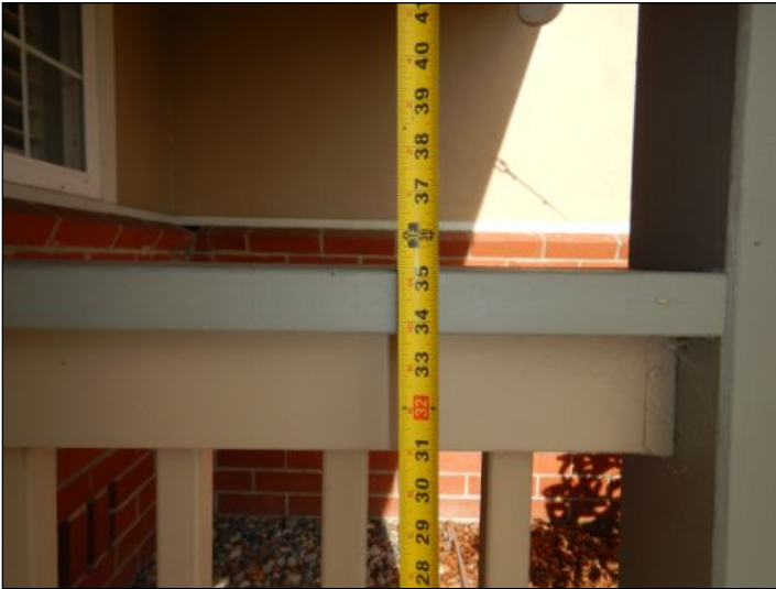
Railing height at the Front Porch of the Main House was below the current standard of 42 inches [2][5]
