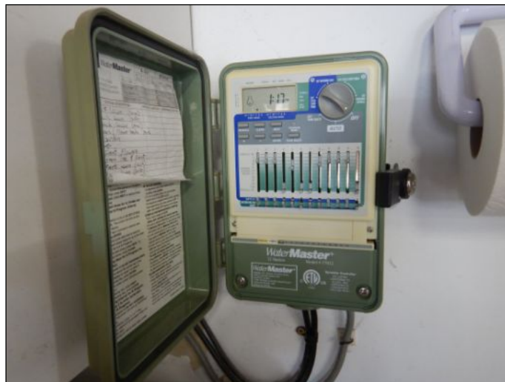
Control Box for the Irrigation System
