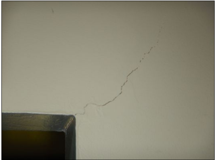
Common cracks in the Walls, consistent with normal home settlement, were noted [1]
