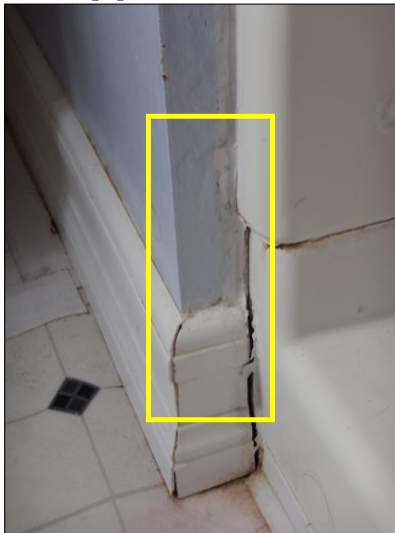
Wall at the Shower in the Master Bathroom had moisture damage; area appeared to be dry at the time of the inspection [2]
