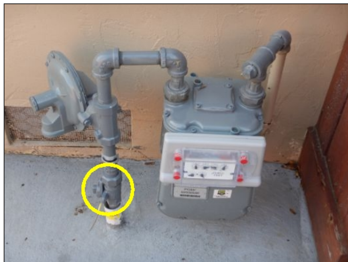
Natural Gas Shut-off valve
