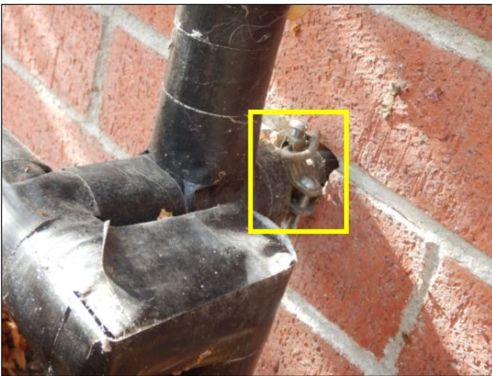
Bonding Wire for the Main Water Line
