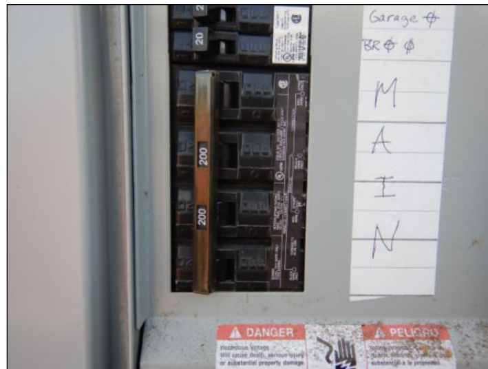
Electrical Service Disconnect
