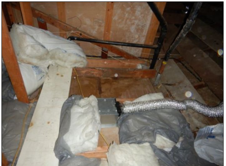
Gaps in the Insulation noted above the Half Bathroom [2]
