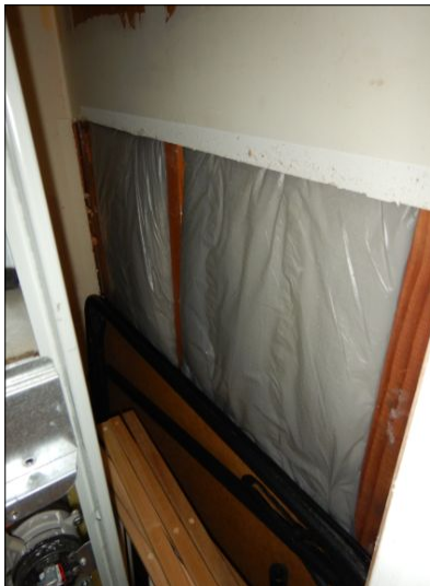
Enclosure Wall was missing Drywall [2]
