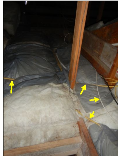
Exposed wire in the Closet of the Master Bedroom below 8 feet and subject to damage [2][4] Unprotected wires were noted within 6 feet of the Attic Access [2][5]
