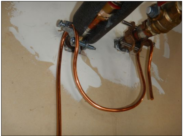
Bonding Wire at the Water Heater
