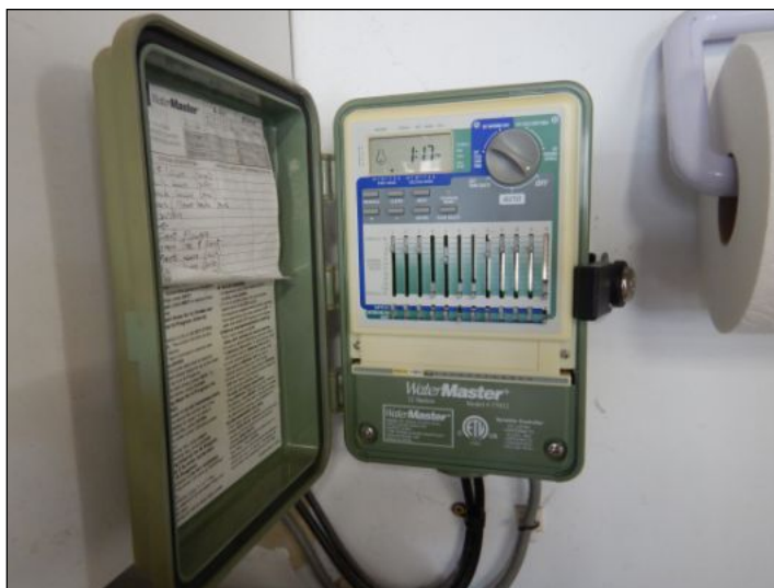
Control Box for the Irrigation System
