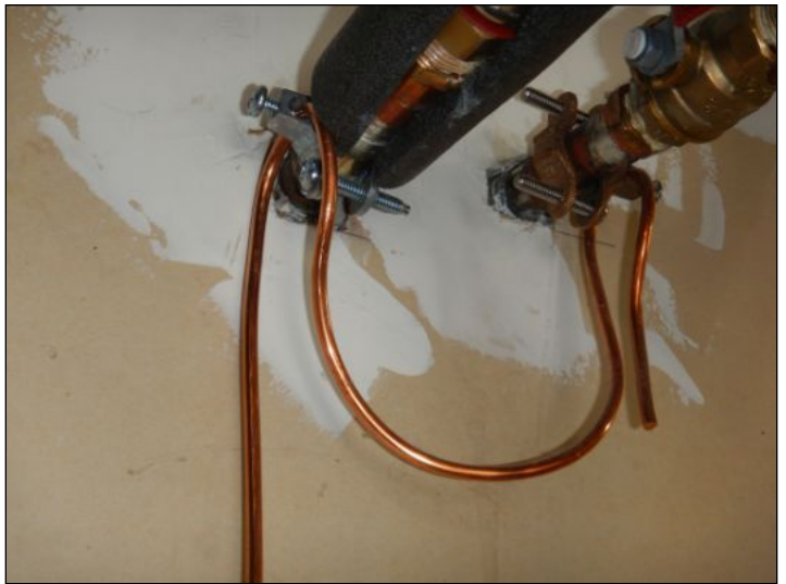
Bonding Wire at the Water Heater
