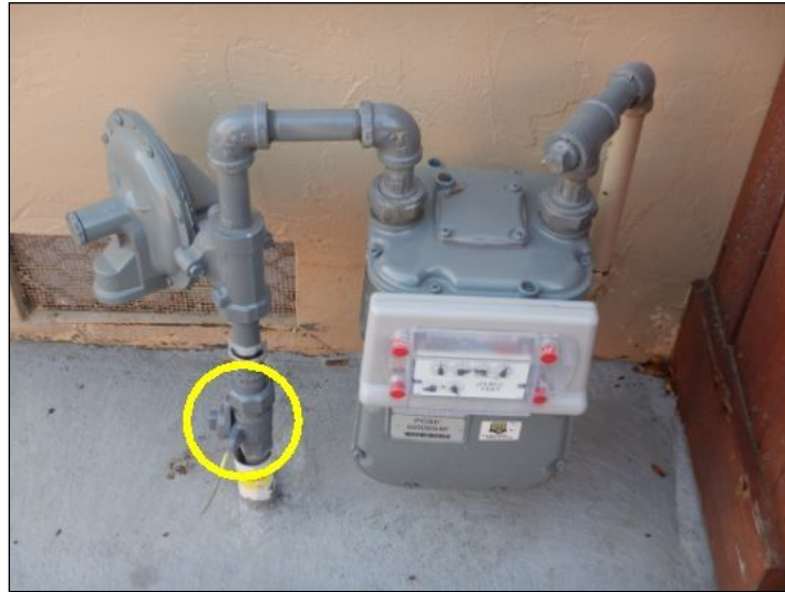
Natural Gas Shut-off valve
