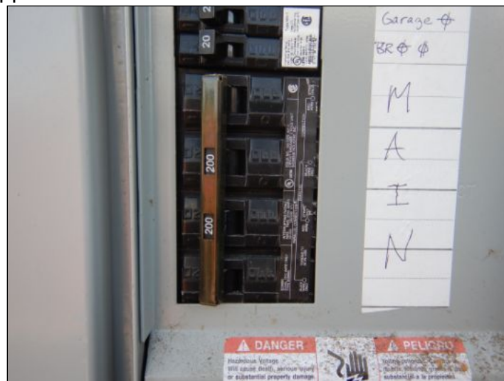
Electrical Service Disconnect
