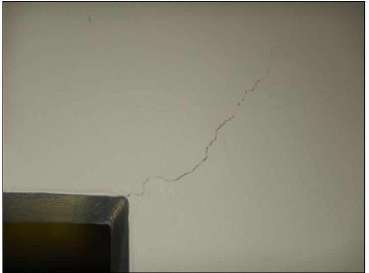
Common cracks in the Walls, consistent with normal building settlement, were noted [1]
