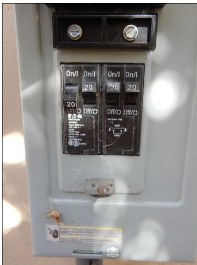
Breakers were not clearly labeled in the Electrical Sub Panel [5]
