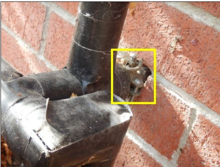
Bonding Wire for the Main Water Line
