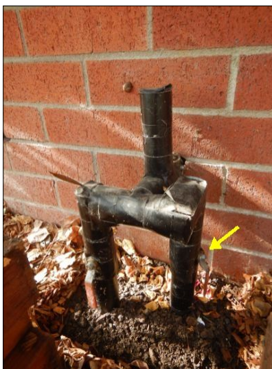
Shutoff Valve for the Main Water Line
